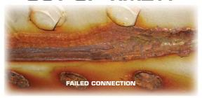
If crevice corrosion and pack rust are affecting the integrity of your structures, the Termarust anti-corrosive coating system is the long-term solution.
