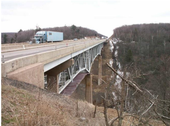
Bridge was built in the 1970’s
