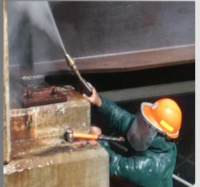
Here, SSPC SP12 WJ4-NV2 surface preparation was effortlessly achieved without negative air containment using a 480 bar, 22 liters per minute hot water pressure wash and Chlor\*Rid. Once dry, **bearings**, **beam ends and lattice joints** surfaces are ready for Zone Painting with Termarust Technologies HR CSA products. *Finally!* A pragmatic way to stop rust bleeding on steel joints and connections!
