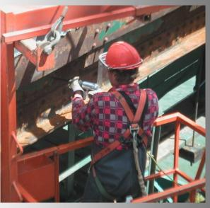
HR CSA TR2200HS penetrant/sealer and TR2100 primer/topcoat have freed corrosion-frozen bearings, stopped pack rust and crevice corrosion, and protected flat surface areas from corroding for decades. [See Case Studies.]
