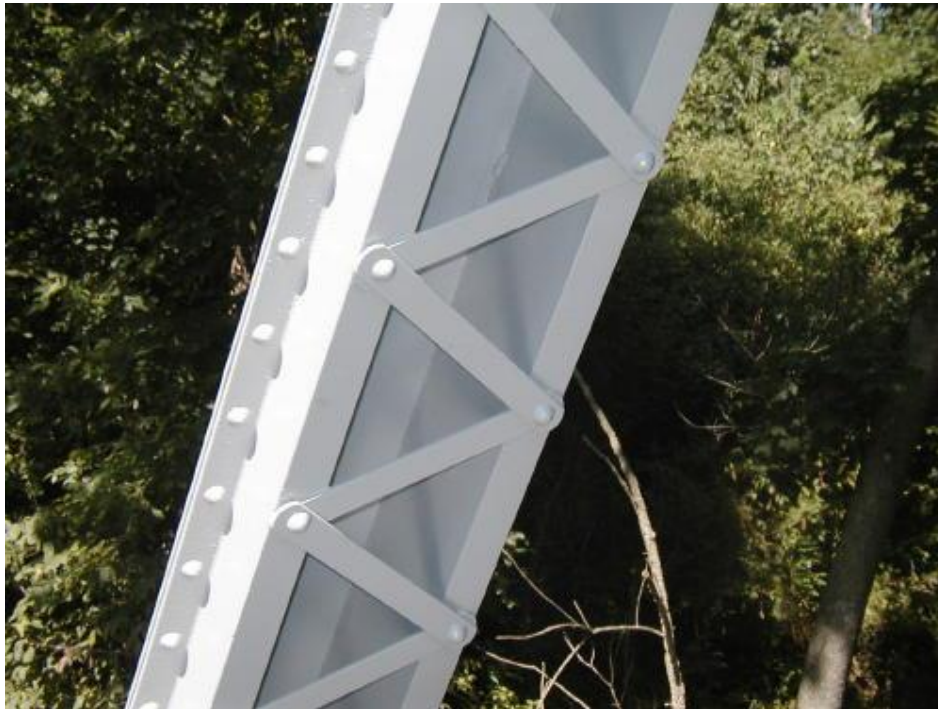
Photo 18 – Painting completed. (see Photo 21)
