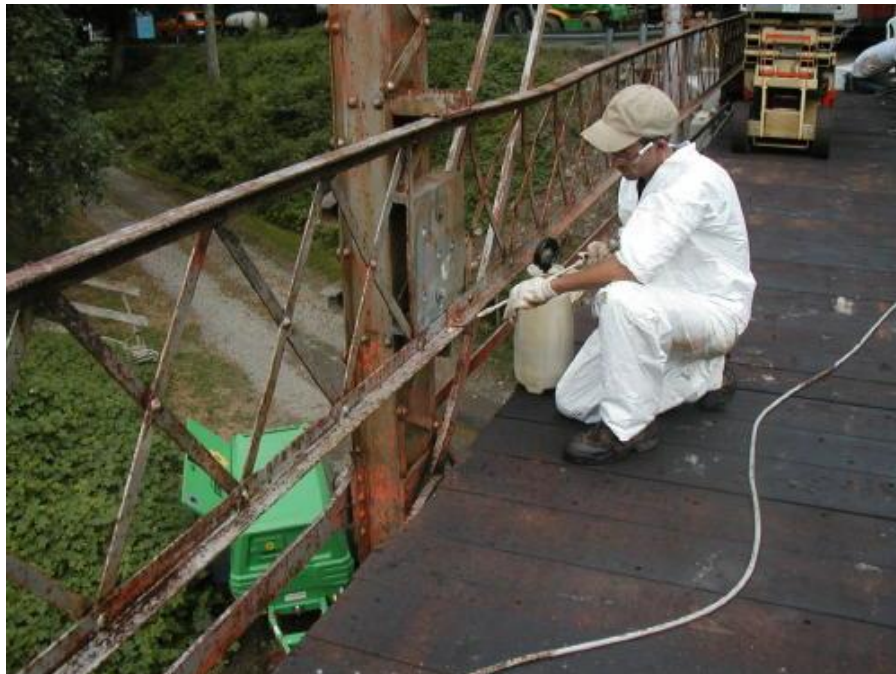
Photo 15 – Applying TR2200 Penetrant to connections.
