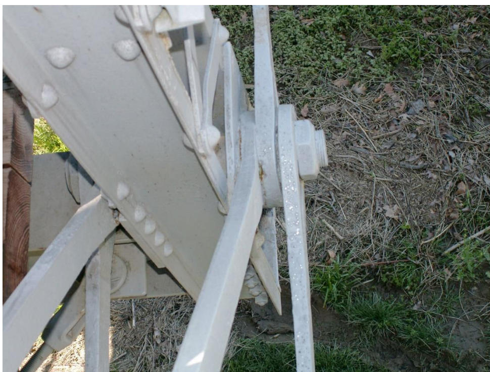
Photo 24 – 20 Months after painting – corrosion in connection has been stopped.
