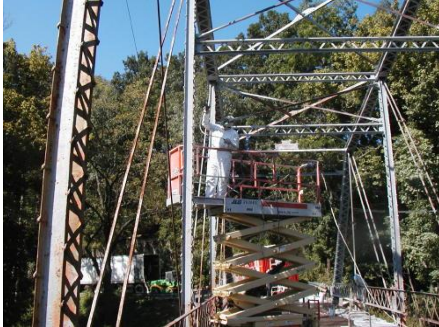
Photo 17 – Painting the bridge from two scissor lifts.
