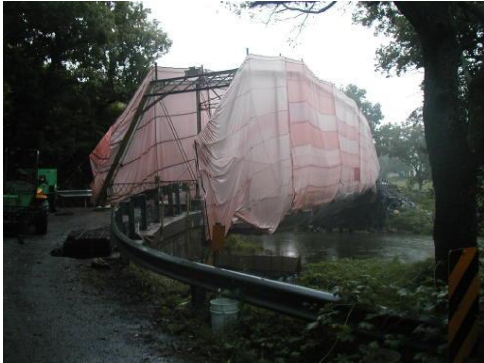
Photo 5 – Tarps for containment for pressure washing
