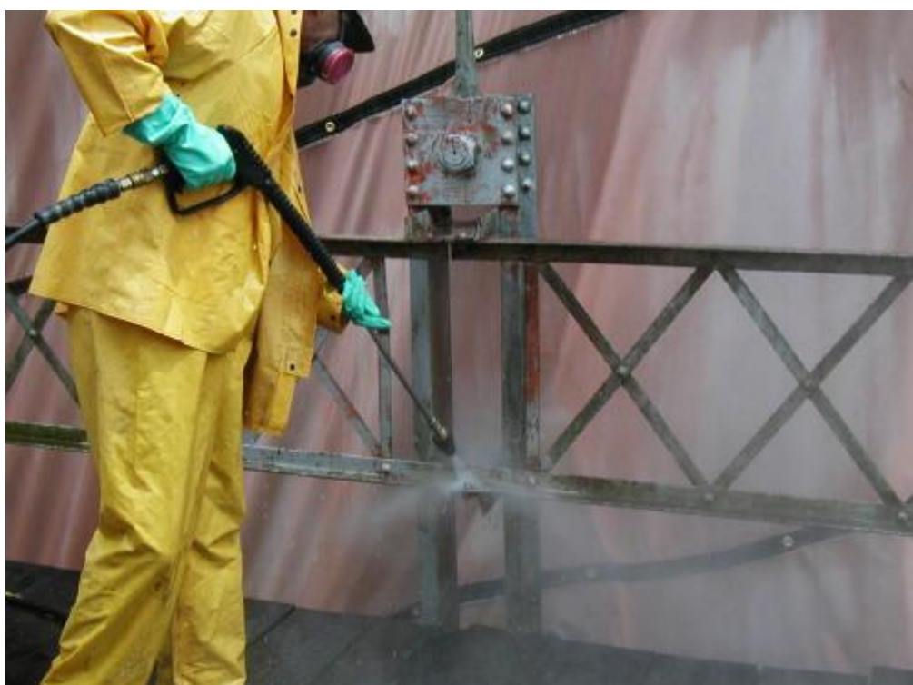
Photo 8 – 5,000 psi pressure washing, standoff distance less than 6”.
