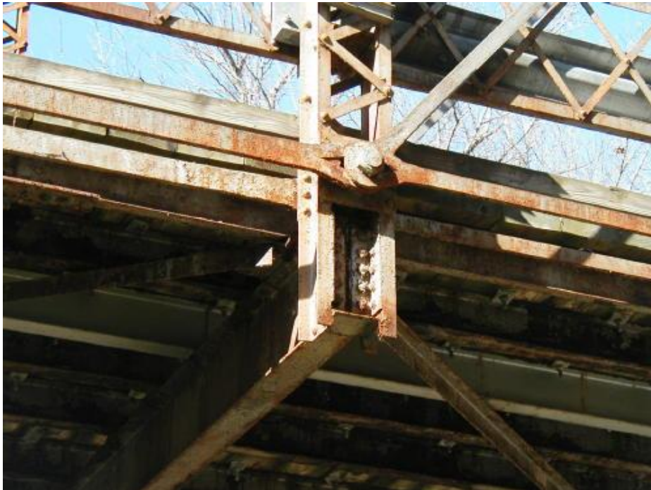
Photo 2 – Bridge in 2004. (see Photo 26)
