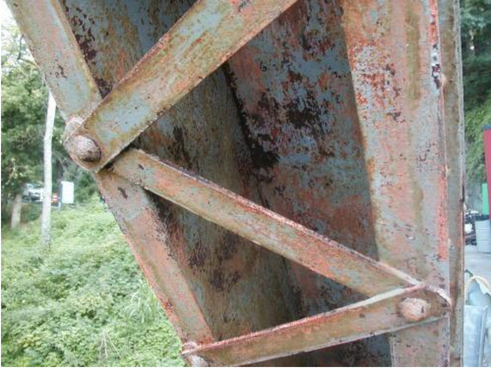
Photo 9 – Truss member cleaned by pressure washing, ready for painting.
