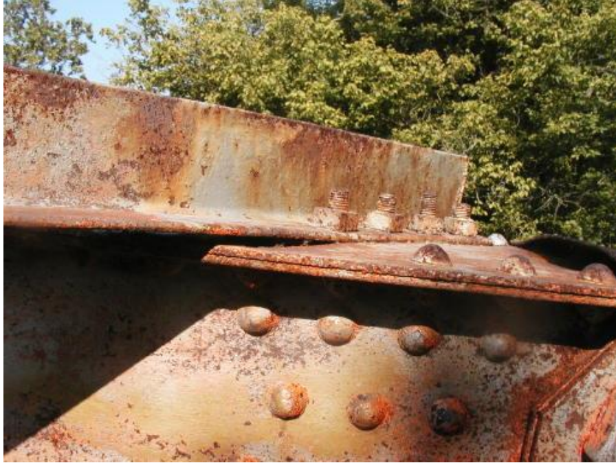
Photo 13 – Top of portal frame cleaned and ready for painting
