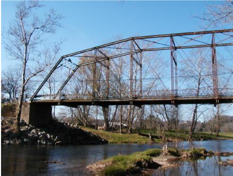
Photo 1 – Bridge in 2004, before painting.
