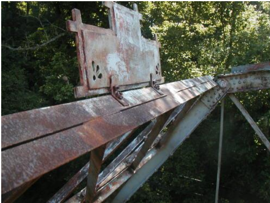
Photo 12 – Top of portal truss cleaned and ready for painting.
