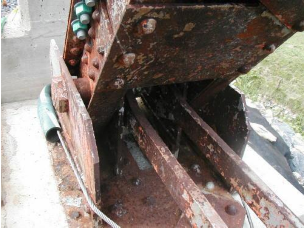
Photo 11 – Pin/truss assembly cleaned and ready for painting.
