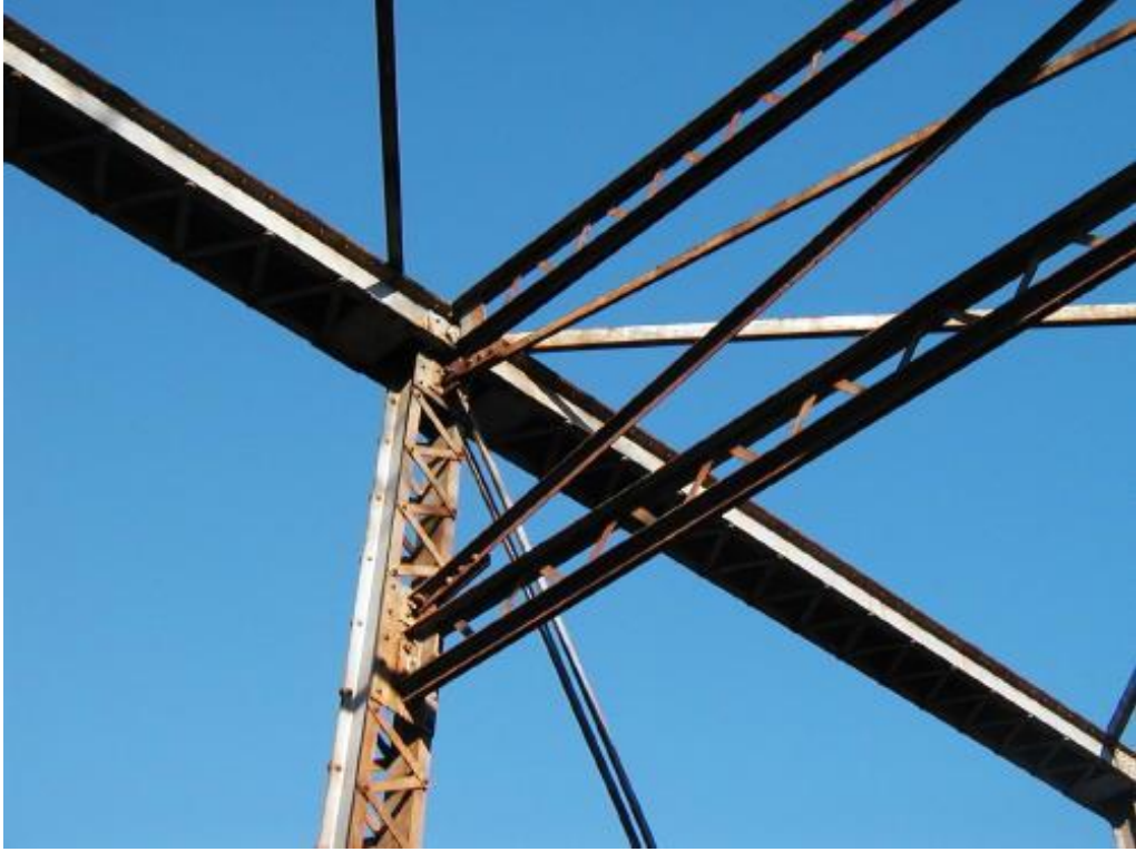
Photo 3 – Bridge in 2004. (see Photo 20)
