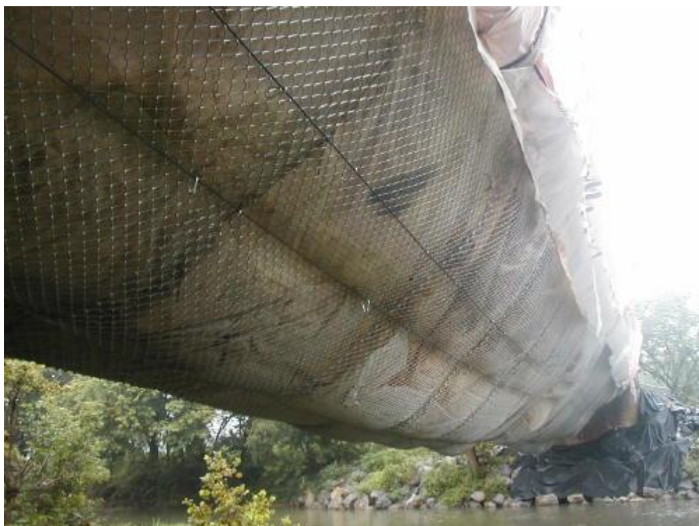
Photo 7 – Underside of containment.
