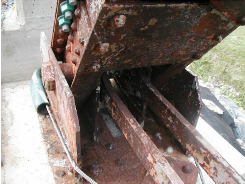
Photo 11 Pin/truss assembly cleaned and ready for painting.
