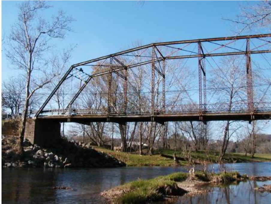
Photo 1 Bridge in 2004, before painting.
