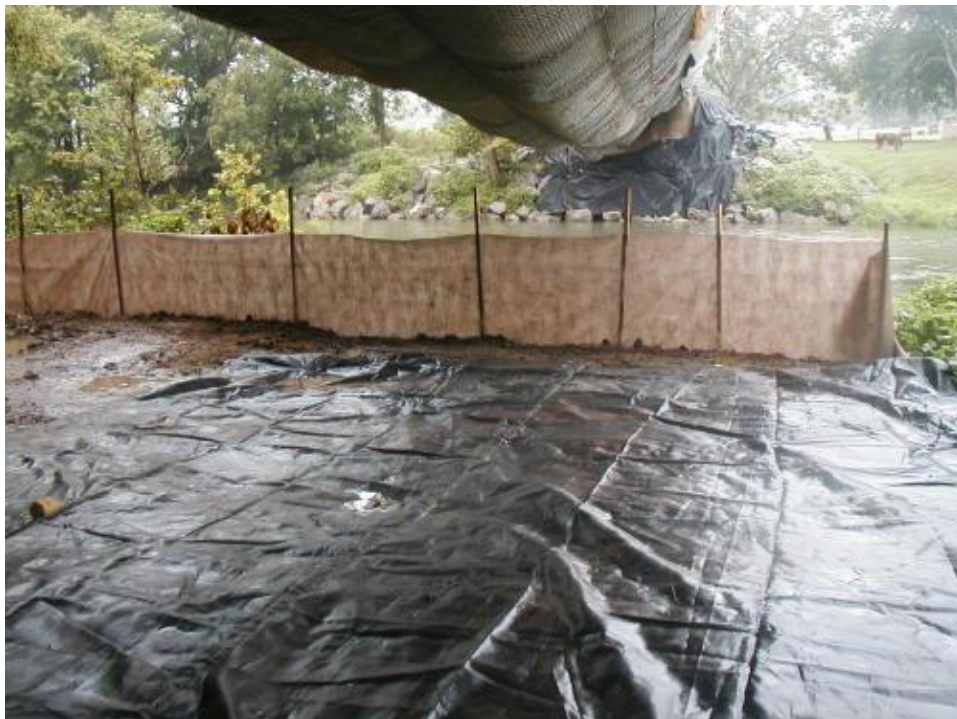
Photo 6 Flow-through tarp and filter fence contain paint chips.
