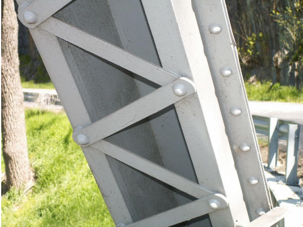
Photo 21 coating has been in service for 12 years .. (see Photos 9 and 18).
