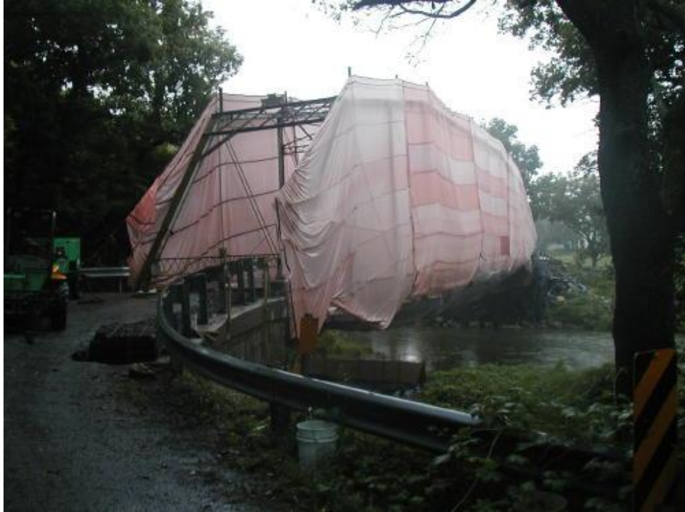
Photo 5 Tarps for containment for pressure washing
