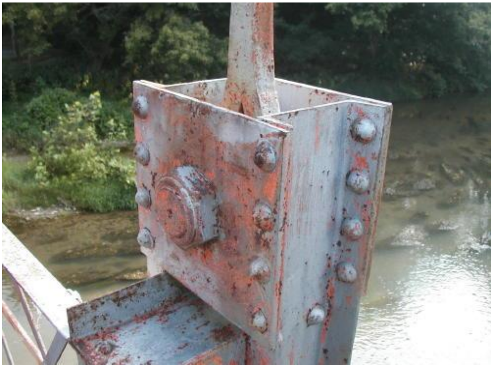
Photo 10 Bottom of tie rod assembly cleaned and ready for painting. (see Photo 25)
