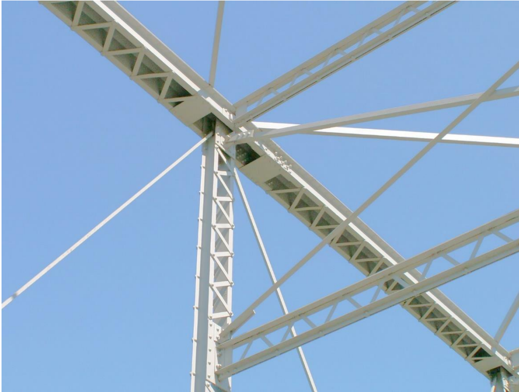
Photo 20 coating has been in service for 12 years . (see Photo 3)
