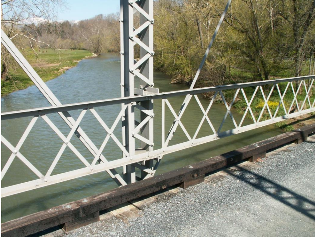
Photo 19 coating has been in service for 12 years . (see Photo 16)
