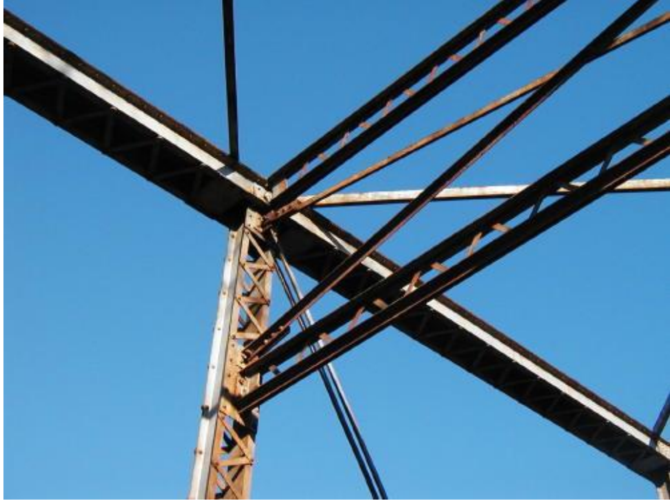
Photo 3 Bridge in 2004. (see Photo 20)
