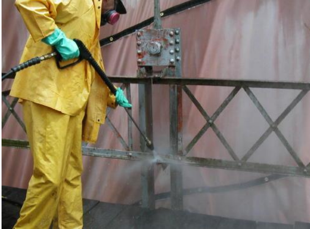
Photo 8 5,000 psi pressure washing, standoff distance less than 4 inches.
