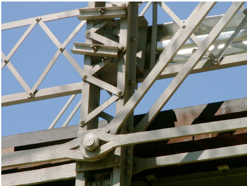
Photo 26 coating has been in service for 12 years . (see Photo 2)
