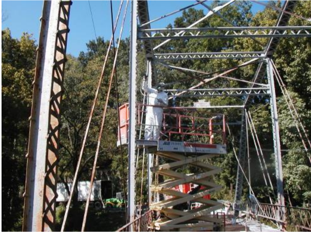
Photo 17 Painting the bridge from two scissor lifts.
