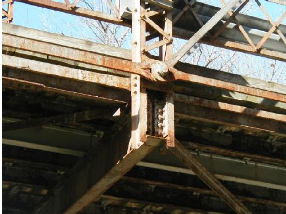
Photo 2 Bridge in 2004. (see Photo 26)
