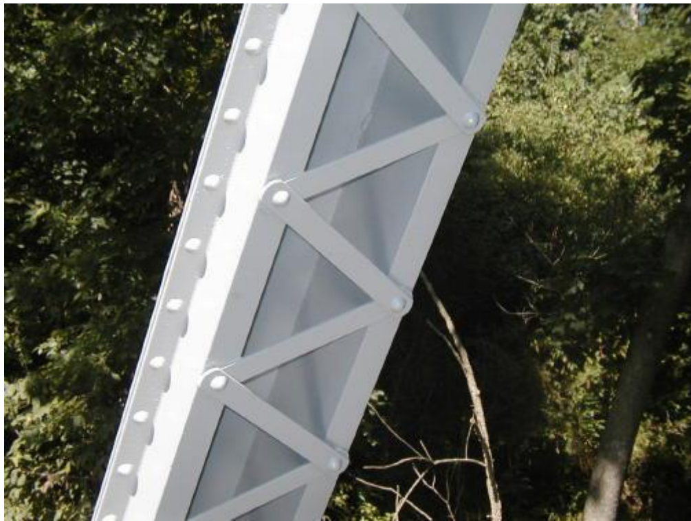
Photo 18 Painting completed. (see Photo 21)
