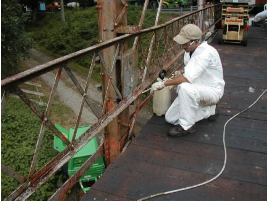
Photo 15 Applying TR2200HS Penetrant/Sealer to connections.
