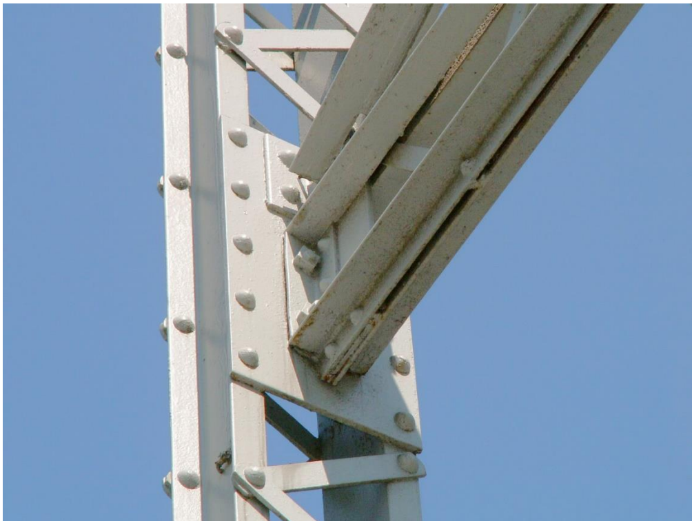
Photo 22 coating has been in service for 12 years . (see Photos 3 and 20)
