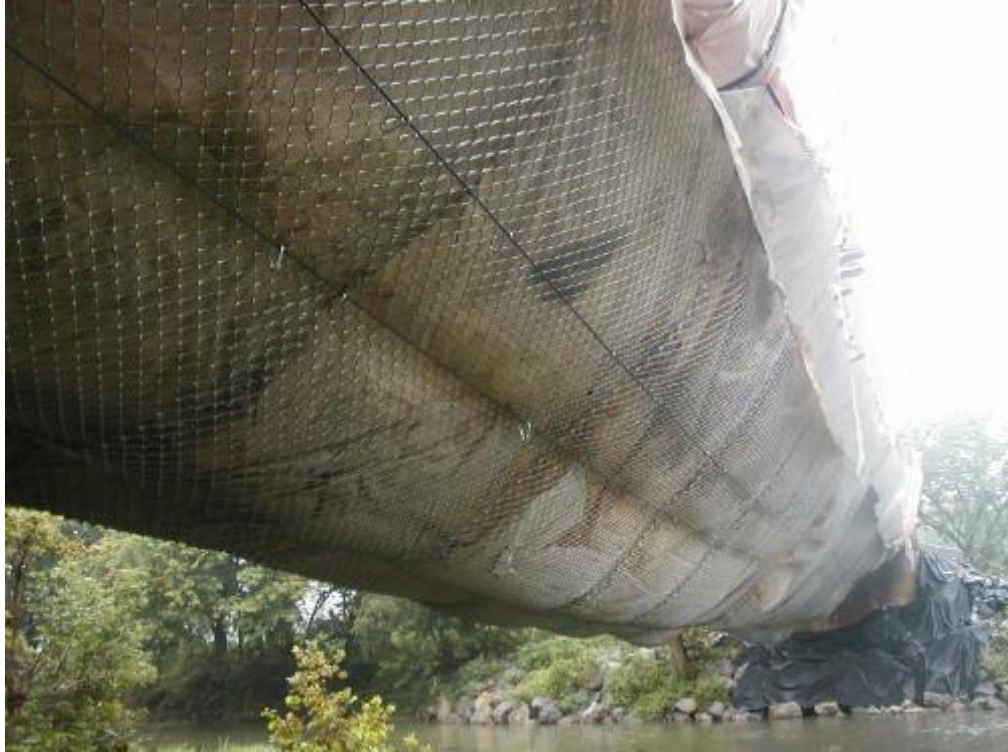
Photo 7 Underside of containment.
