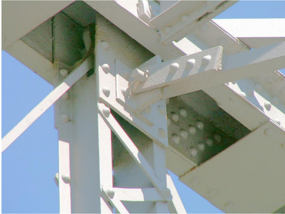
Photo 23 coating has been in service for 12 years . (see Photos 3 and 20)
