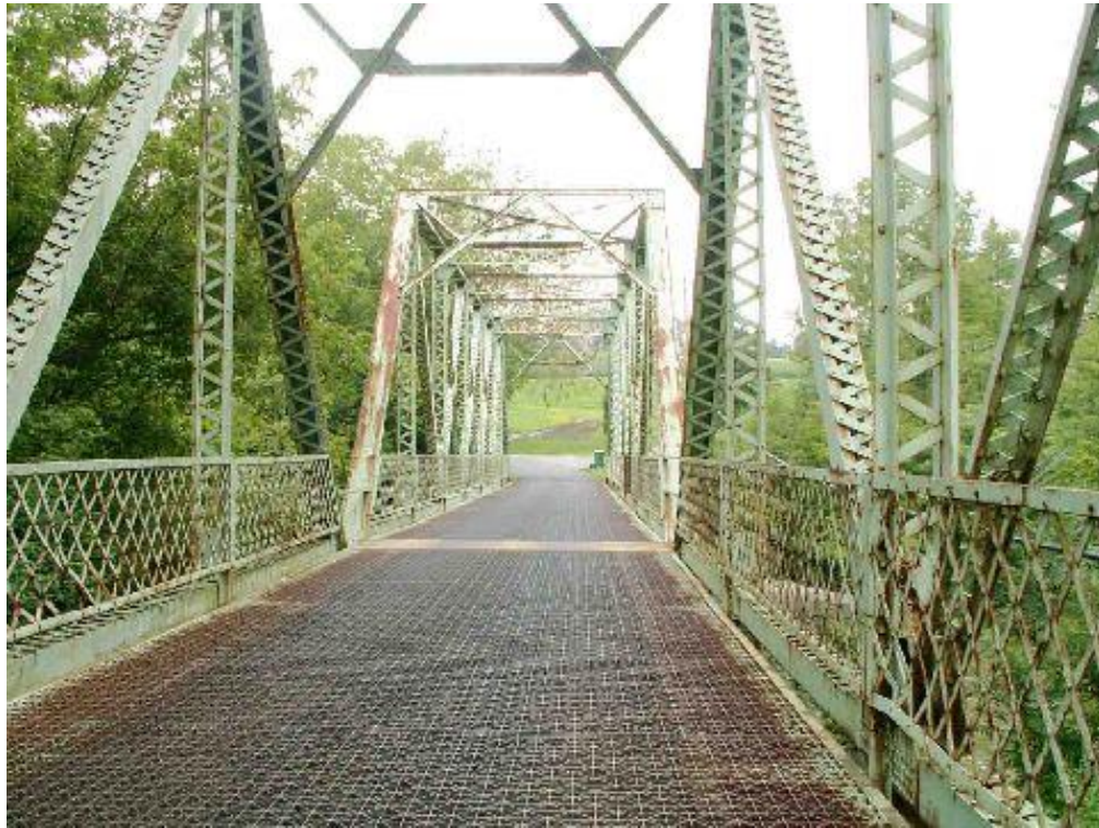
Photo 1 – Bridge before cleaning and coating with the Termarust system.
