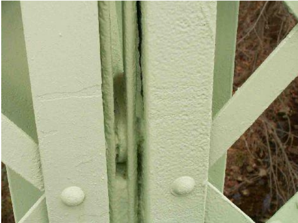
Photo 13 – Close-up of a complex connection (See Photo 7)
