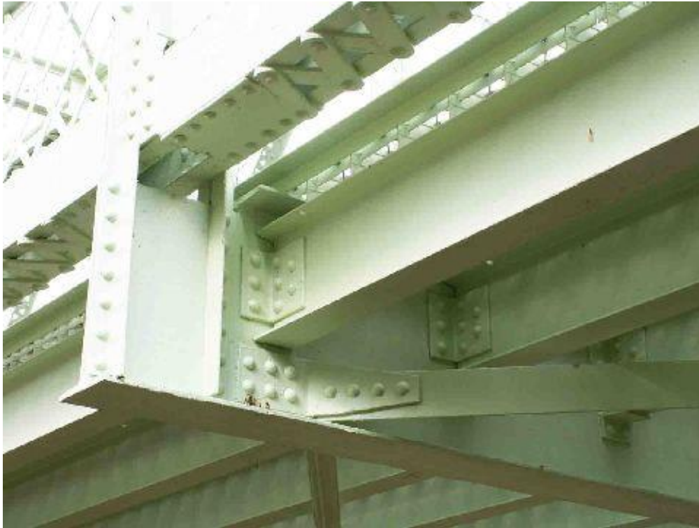
Photo 15 – Coating has been completed (See Photos 8 and 9)
