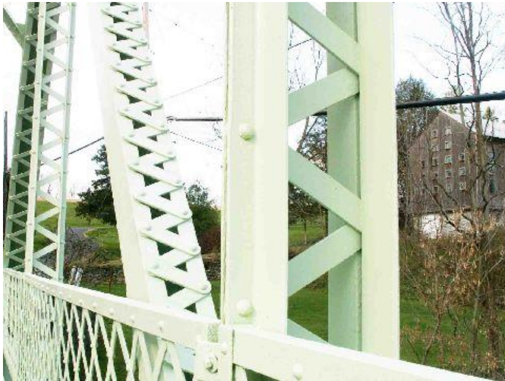
Photo 12 – Bridge members have been coated with the Termarust system
