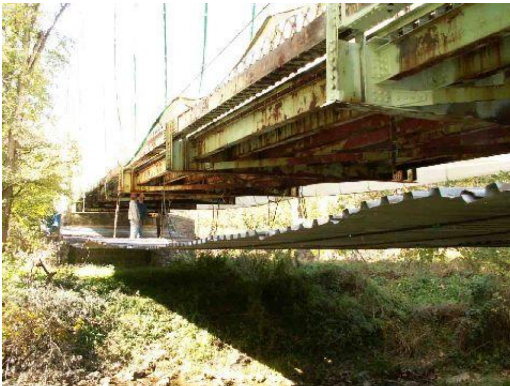
Photo 8 – Work platform – Containment tarps were removed after pressure washing.
