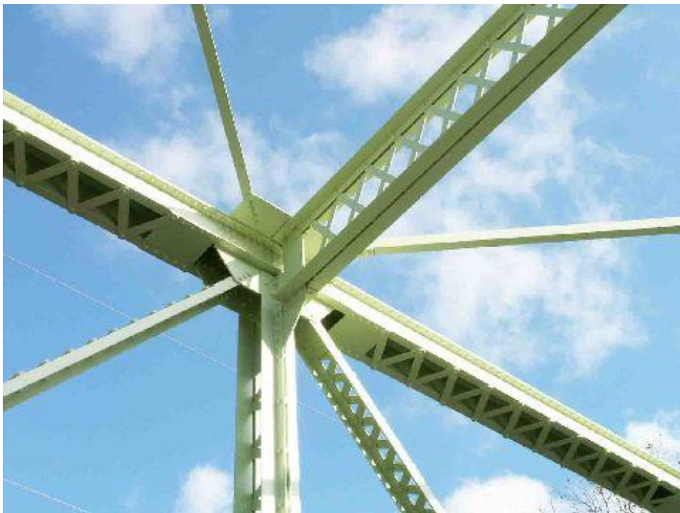
Photo 14 – Coating has been completed (See Photo 2)
