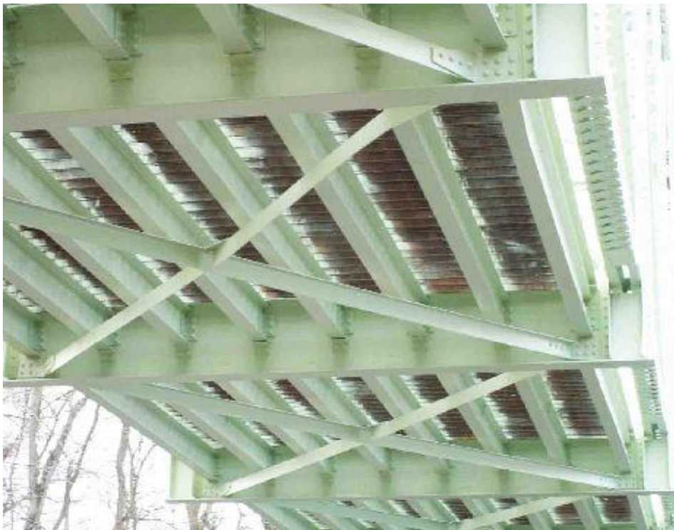
Photo 16 – Coating has been completed and corrosion stopped. (See Photos 4, 5 and 10)
