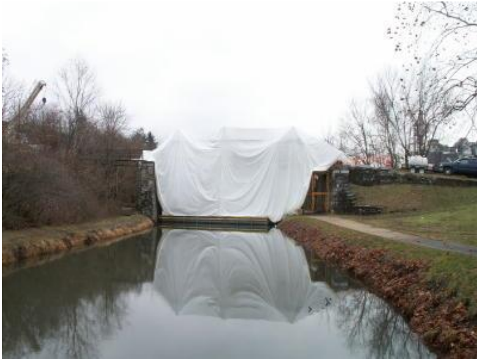
Photo 8 Bridge is covered with a tarp, for cleaning and painting
