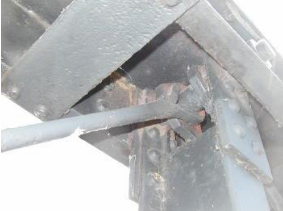
Photo 7 Upper tie-rod and truss connection.
