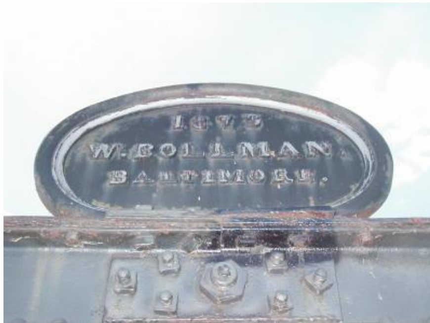
Photo 2 Memorial plaque on bridge: 1879 W. Bollman Baltimore.
