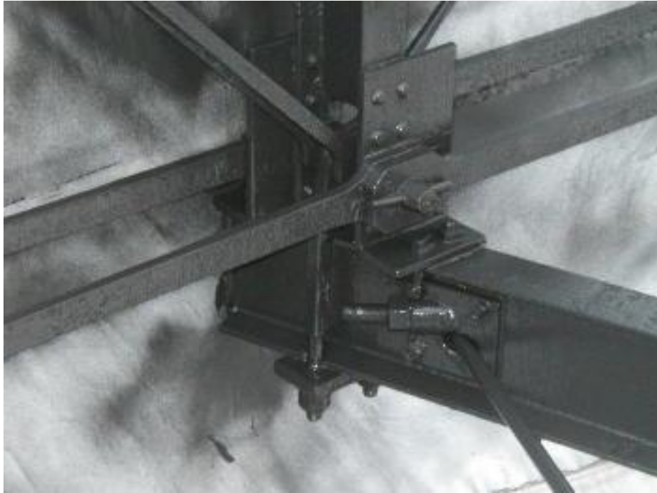
Photo 15 The connection has been coated with the TR2100 Topcoat.
