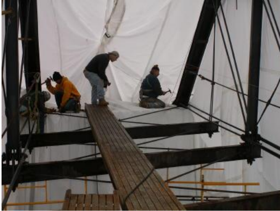
Photo 9 Removing scale rust before pressure washing
