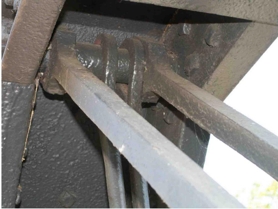
Photo 25 May 12, 2009 Corrosion has been stopped.
