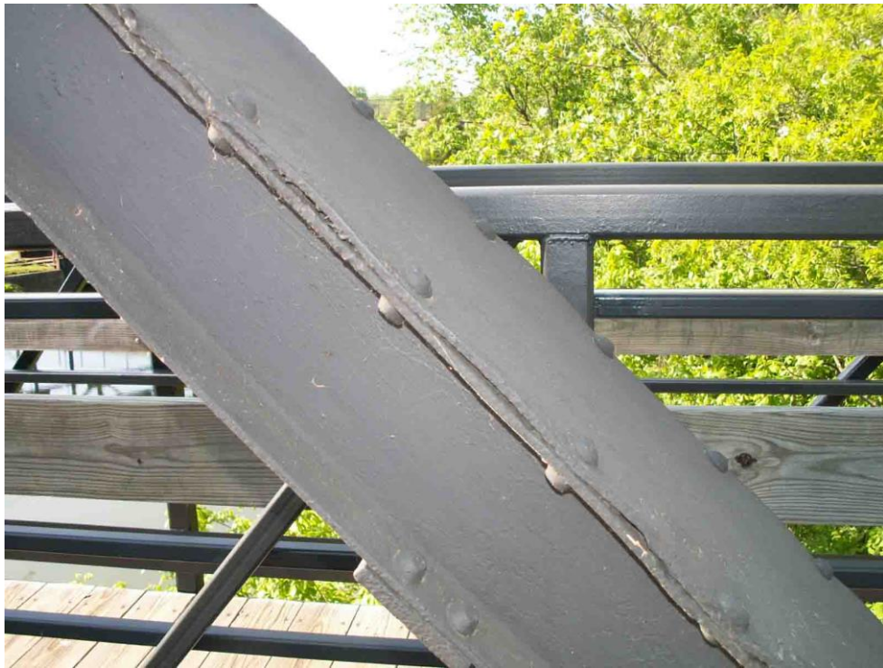
Photo 23 May 12, 2009 Crevice corrosion has been stopped.
