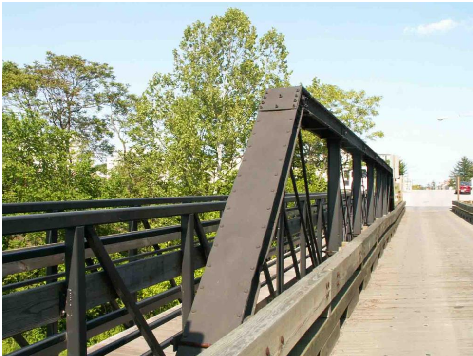
Photo 22 May 12, 2009 No coating or corrosion problems.
