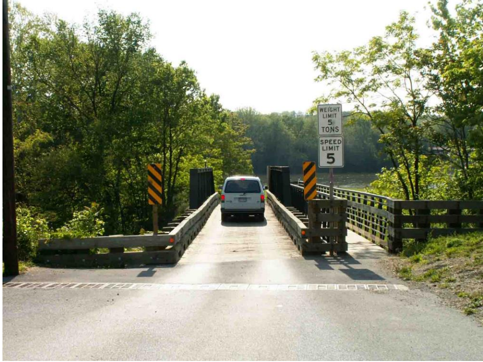
Photo 21 May 12, 2009 View of completed bridge work
