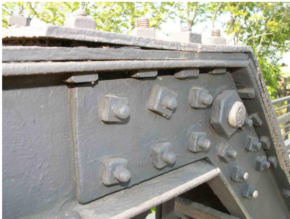
Photo 24 May 12, 2009 Corrosion has been stopped.
