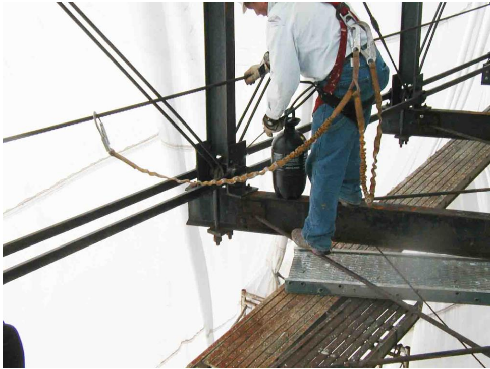
Photo 12 Applying the TR2200 Penetrant into connections.
