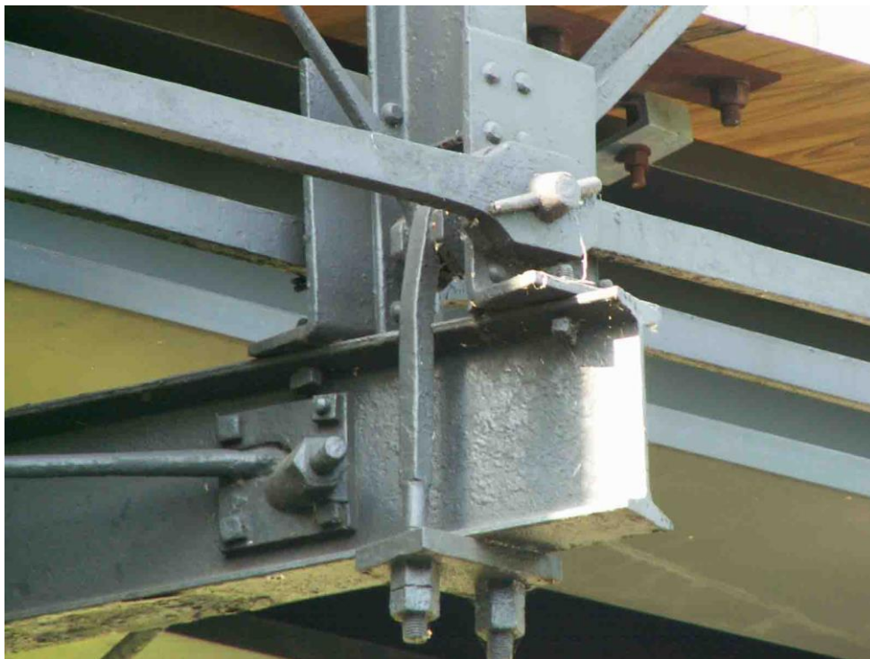
Photo 27 May 12, 2009 No coating or corrosion problems.
