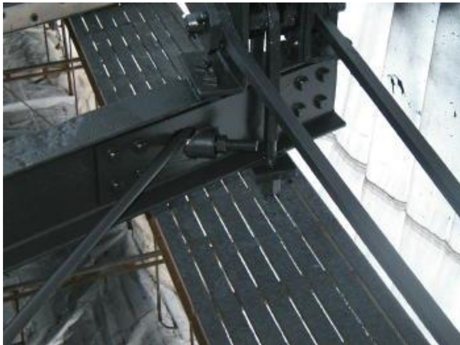
Photo 16 ◆ TR2200 and TR2100 has been applied to the connection ◆ after it was strengthened,
