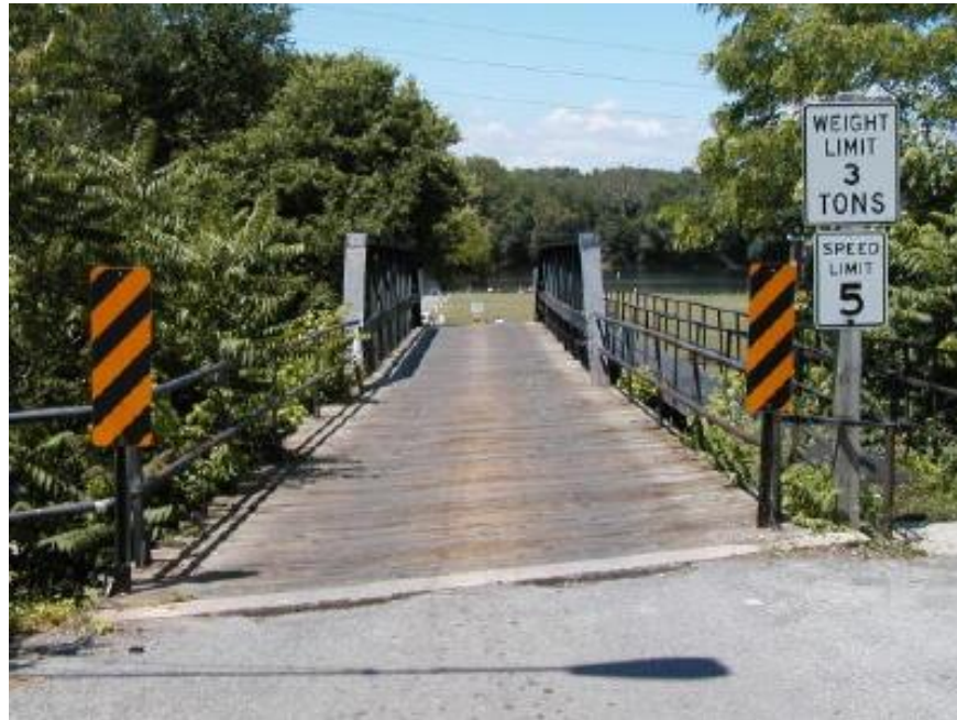
Photo 1 Bridge, and approach span, in 2005, before painting.
