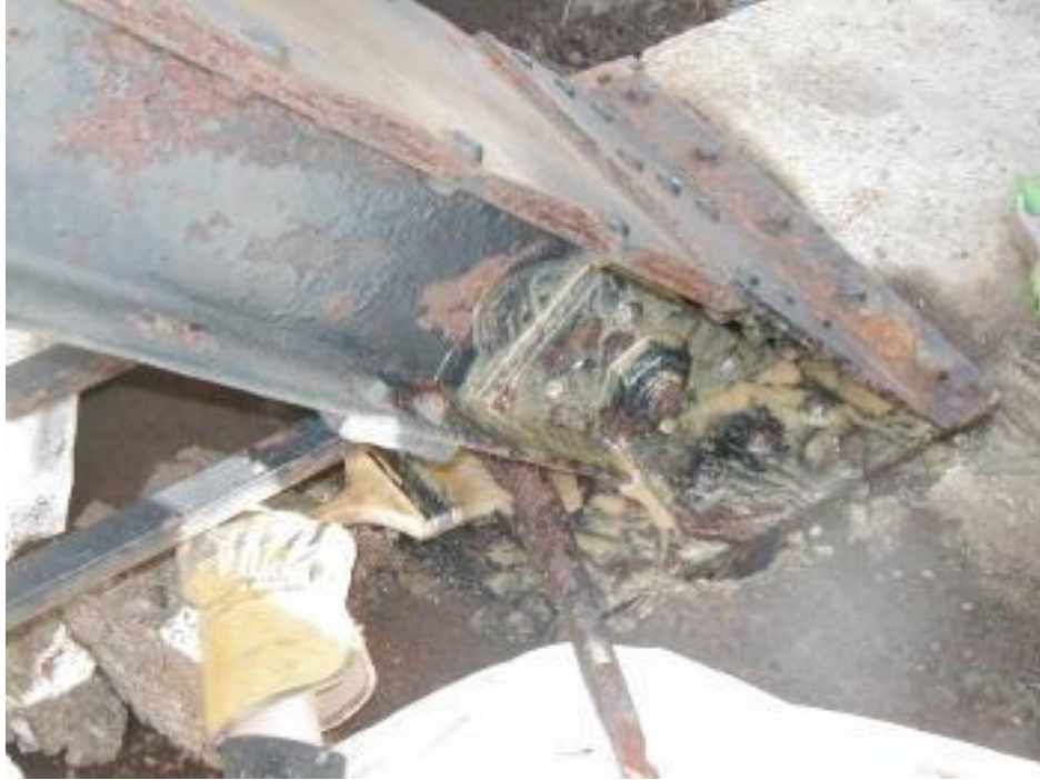
Photo 13 TR2200 Penetrant has been applied to front bearing connection.
