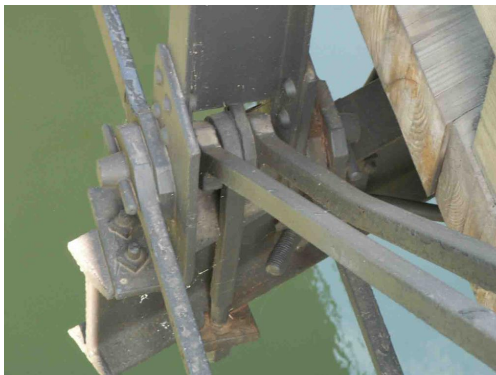
Photo 28 May 12, 2009 No coating or corrosion problems.
