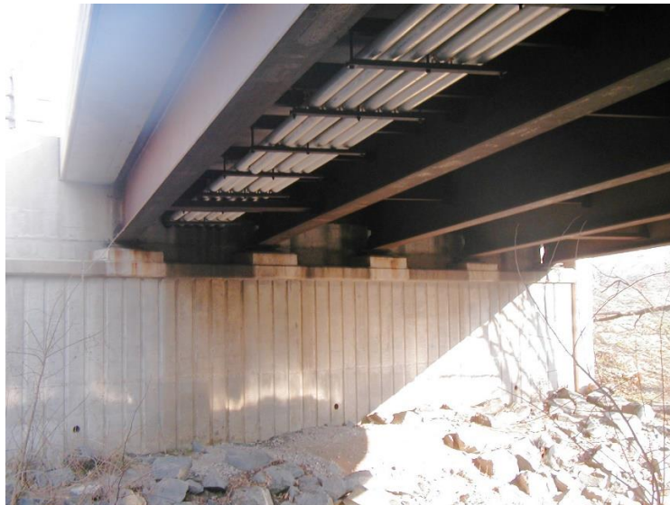
Photo 2 Underside of one of the bridges.
