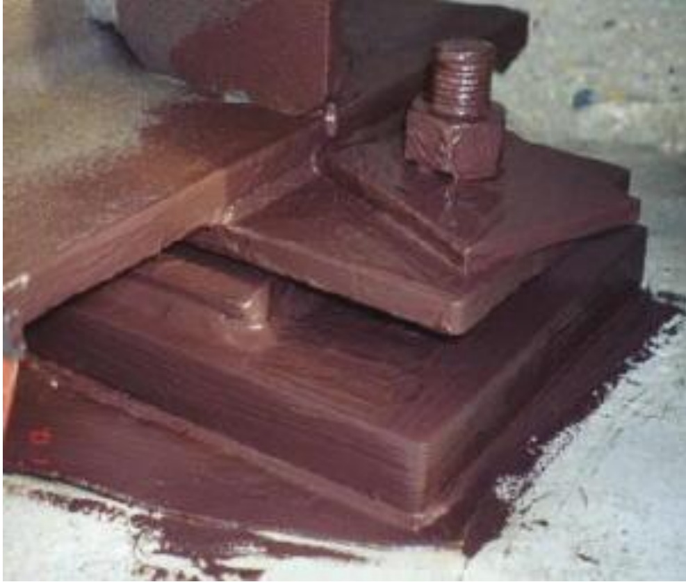
Photo 7 August 2001 after sandblasting and painting with Termarust.
