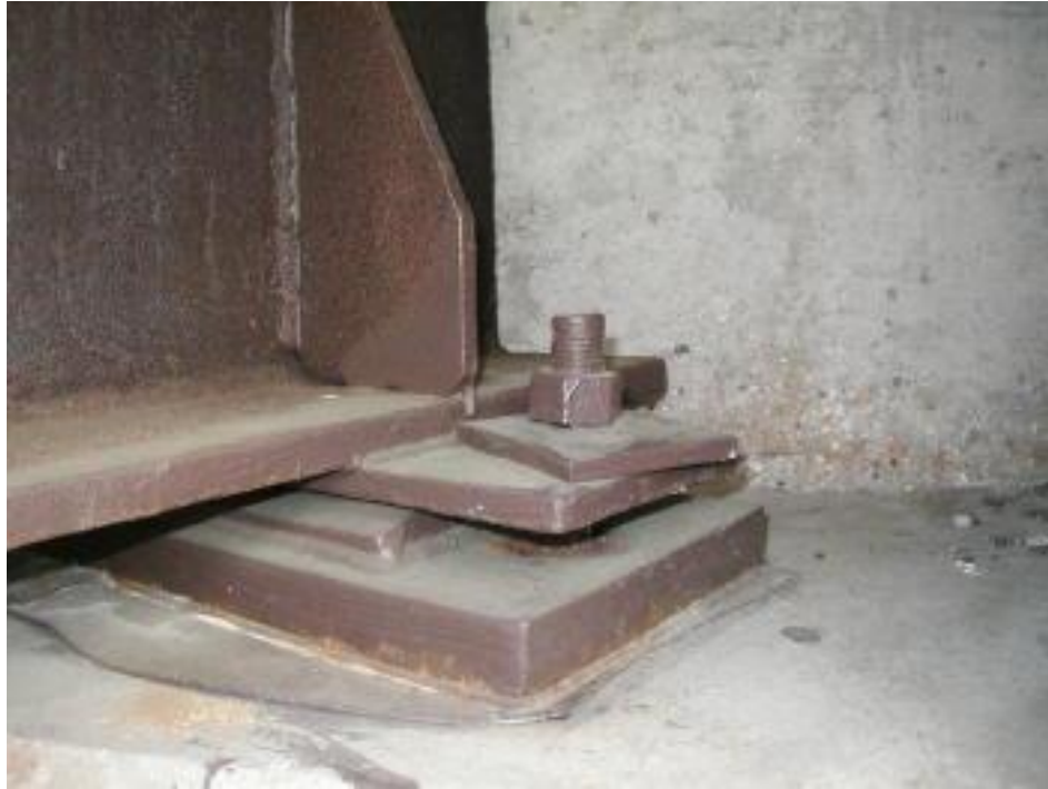
Photo 13 Condition in May 2005, no corrosion of the bearings or anchor bolts.
