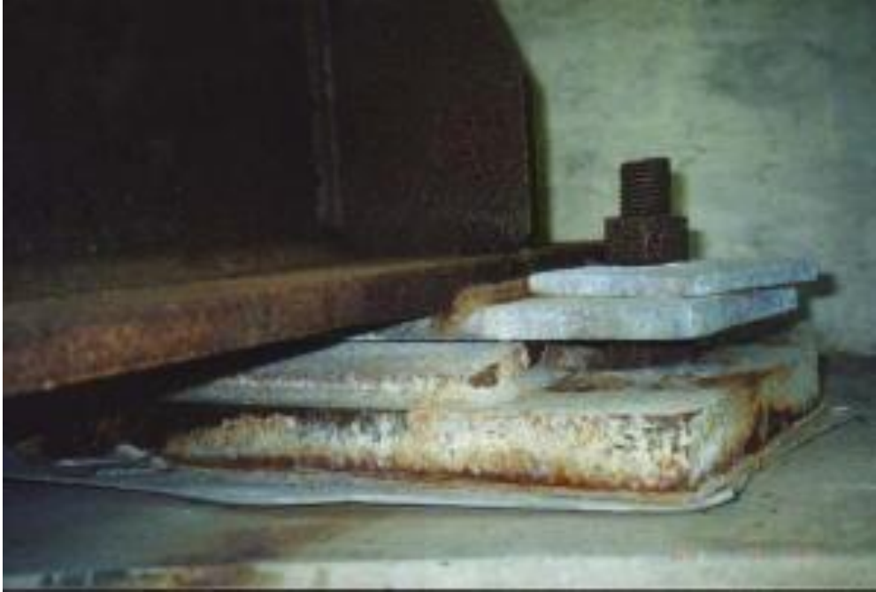
Photo 3 Existing condition of bearings in July 2001.
