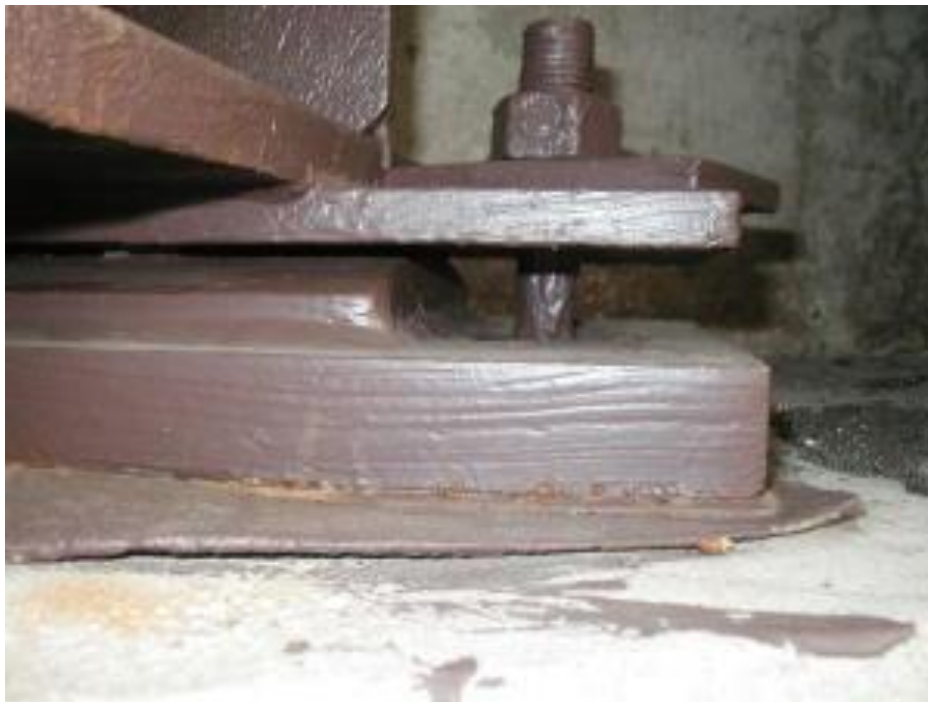
Photo 10 Condition in November 2003, no corrosion after 27 months.
