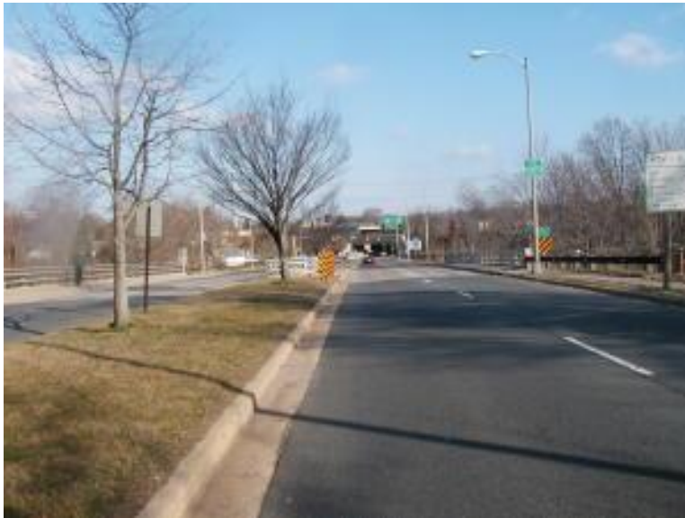
Photo 1 Bridges and the general location.
